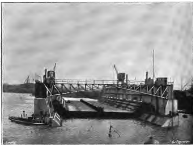
Fig. 514. —Dock Sunk, bringing Centre Pontoon Connection into Upper Position.
